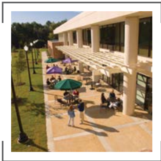
The building was expanded, adding the West Wing, in 2006.
